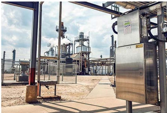
Proper molecular sieve dehydration system operation is critical to operating any natural gas processing or LNG plant. The process hinges on the analyzer that tests the desiccant dryer outlet gas for moisture content. A bad measurement can be a major economic blow or even force a shutdown of the plant. In response to this need, some plant managers are turning to tunable-diode laser (TDL) analyzers. SpectraSensors in Houston, Texas has provided over 90% of installed extractive TDL analyzers.
