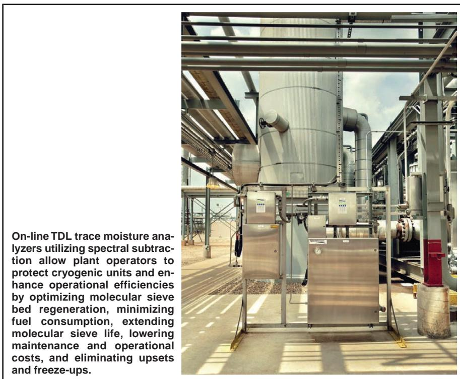
**On-line TDL trace moisture analyzers utilizing spectral subtraction allow plant operators to protect cryogenic units and enhance operational efficiencies by optimizing molecular sieve bed regeneration, minimizing fuel consumption, extending molecular sieve life, lowering maintenance and operational costs, and eliminating upsets and freeze-ups.**
