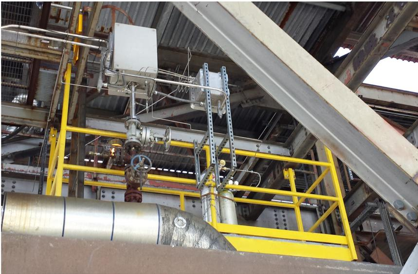
Backside view of the OptoDRS installation on an isolation valve at the sample tap of the gasifier effluent process pipe.
