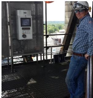
Gasifier installation showing installed Optograf Analyzer.
